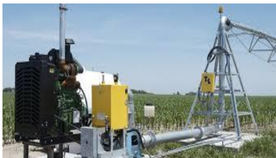
Fig 3 Pump and center of pivot
